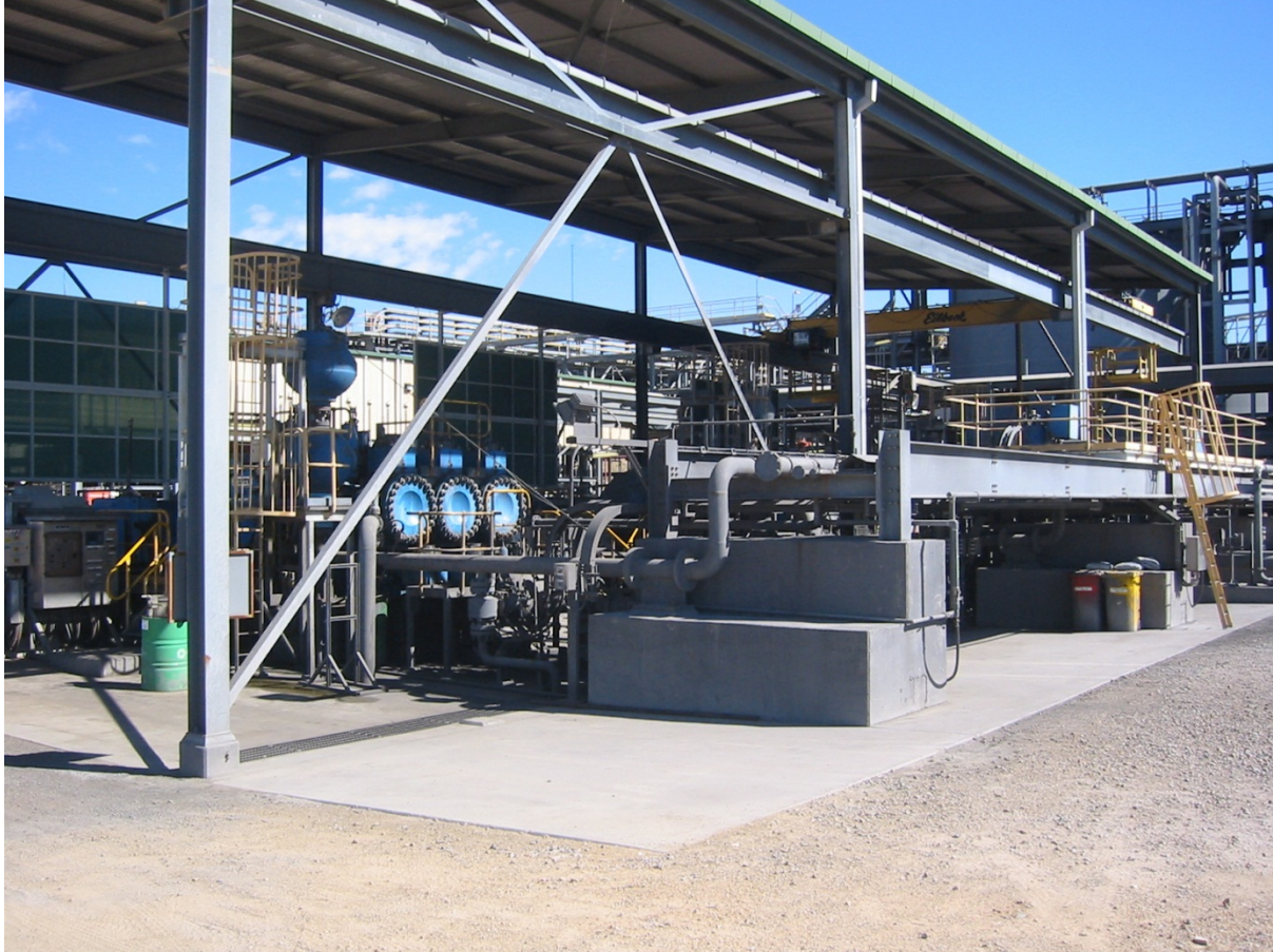
Figure 2 View of Century Pump Station
